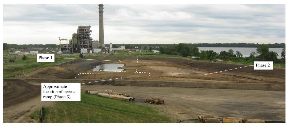
Photo was taken on July 9, 2020, from the west side of the North and South Ash Impoundments looking east, following the completion of removal of the access ramp (Phase 3). Clay was observed at the base of the unit in all locations. Survey information for this phase was taken on July 14, 2020.
