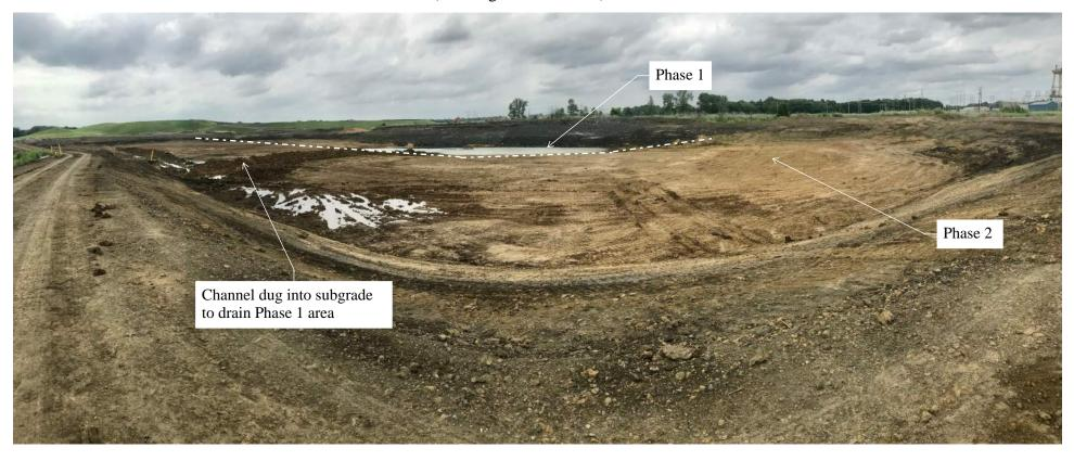
Photo was taken on June 29, 2020, from the south-east corner of the South Ash Impoundment looking west to north, following the completion of CCR removal operations of the South Ash Impoundment. Clay is observed at the base of the unit. Survey information for this phase was taken on July 2, 2020.
