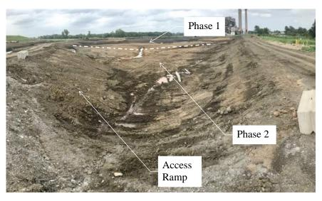
Photos were taken on June 29, 2020, from the west side of the Ash Impoundment looking east and south and north and east, respectively, following the completion of CCR removal operations of the South Ash Impoundment. Clay is observed at the base of the unit. Survey information for this phase was taken on July 2, 2020.
