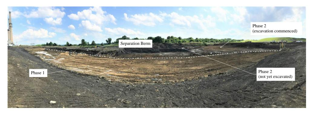
Photo was taken on June 9, 2020, from the west side of the Ash Impoundment looking east and south, following the completion of CCR removal operations of the North Ash Impoundment. Clay is observed at the base of the unit and a portion of the separation berm is observed on the eastern end. Survey information for this phase was taken on June 12, 2020.
