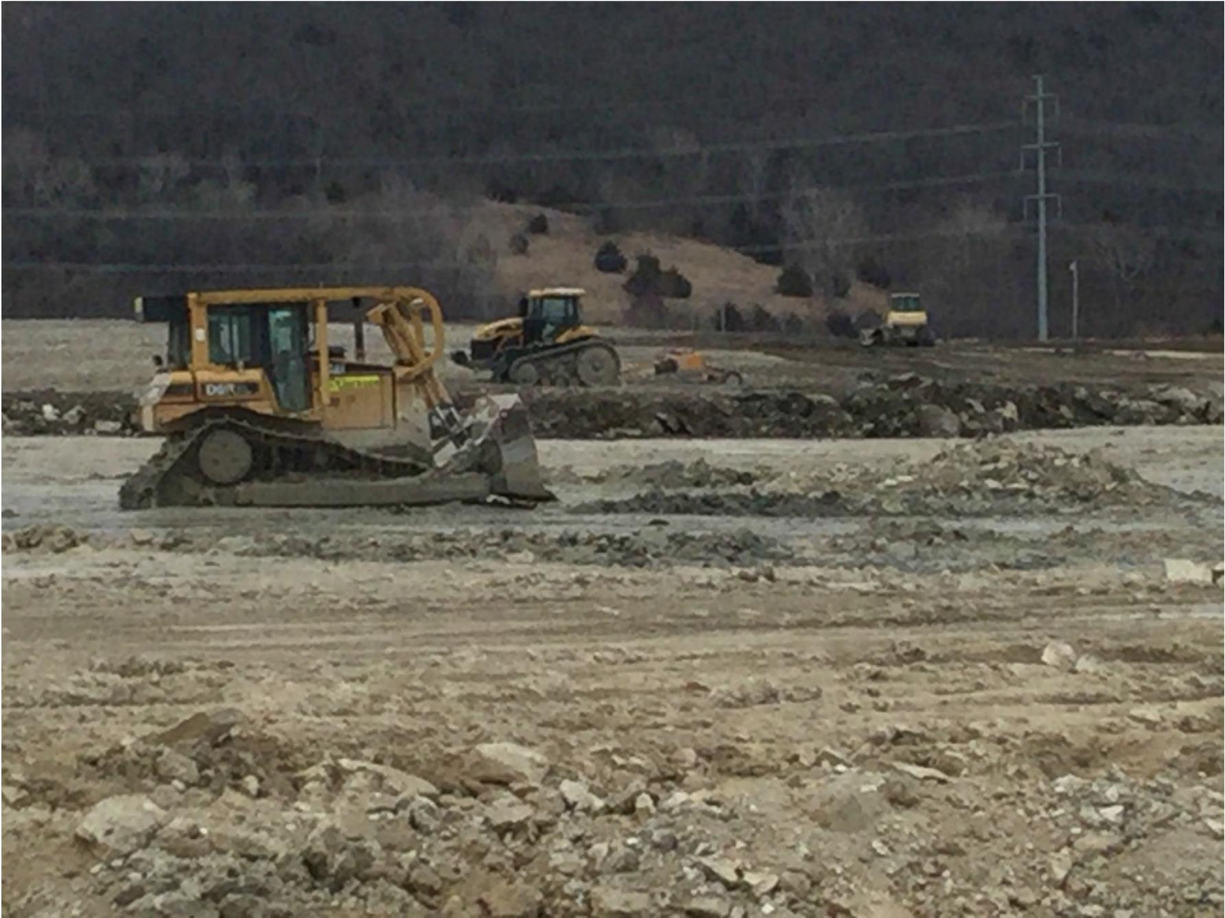
Figure 18: Iatan CCR Landfill – processing excavated ash (looking east)
