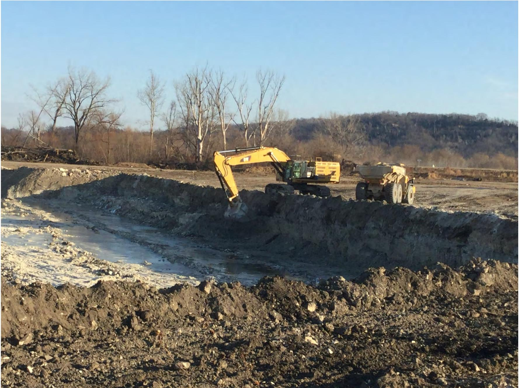
Figure 4: Iatan Ash Impoundment – mechanical excavation from north portion of pond (looking northeast)
