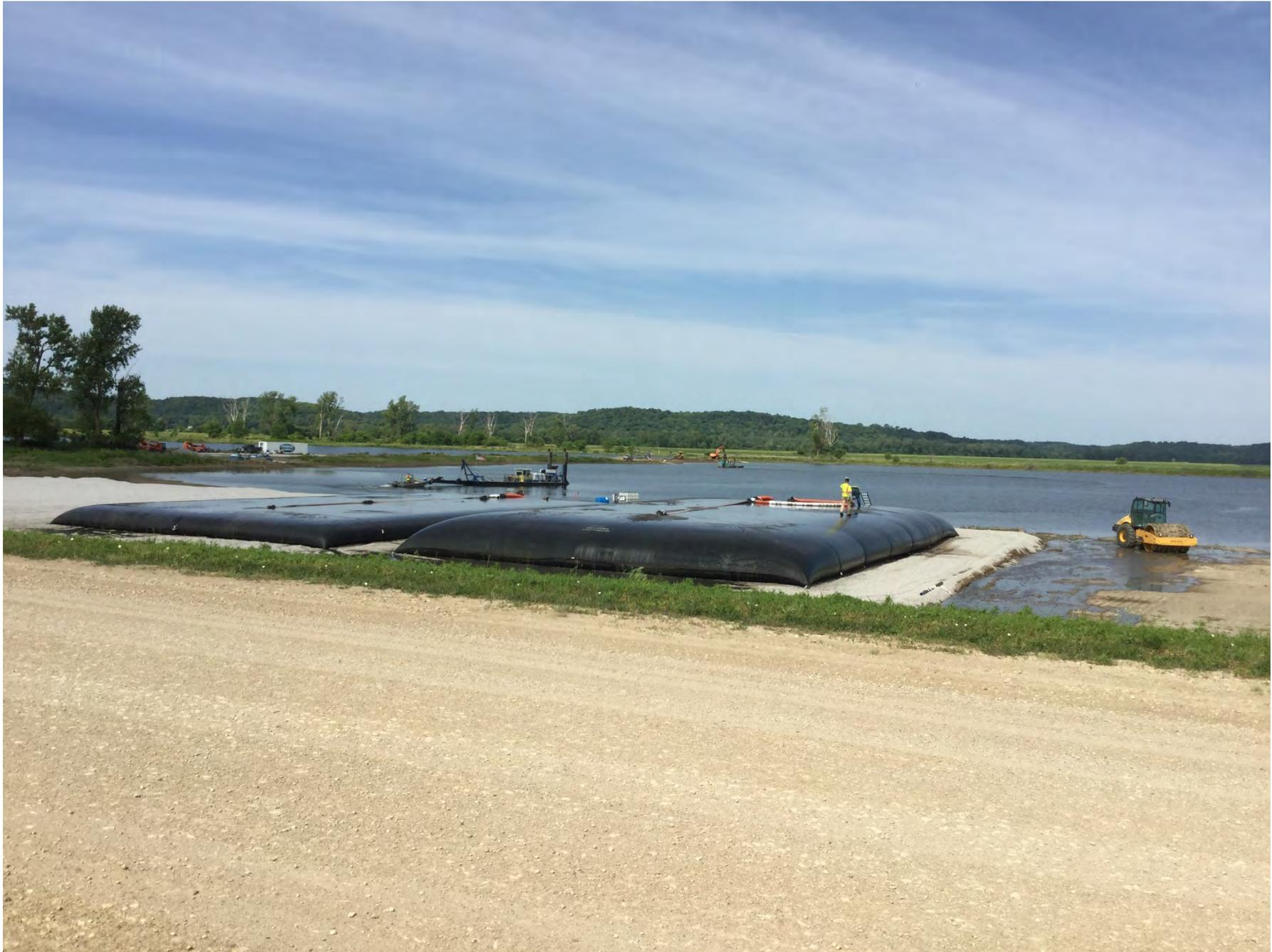
Figure 11: Iatan Ash Impoundment – filling geotextile tubes (east bank looking southwest)
