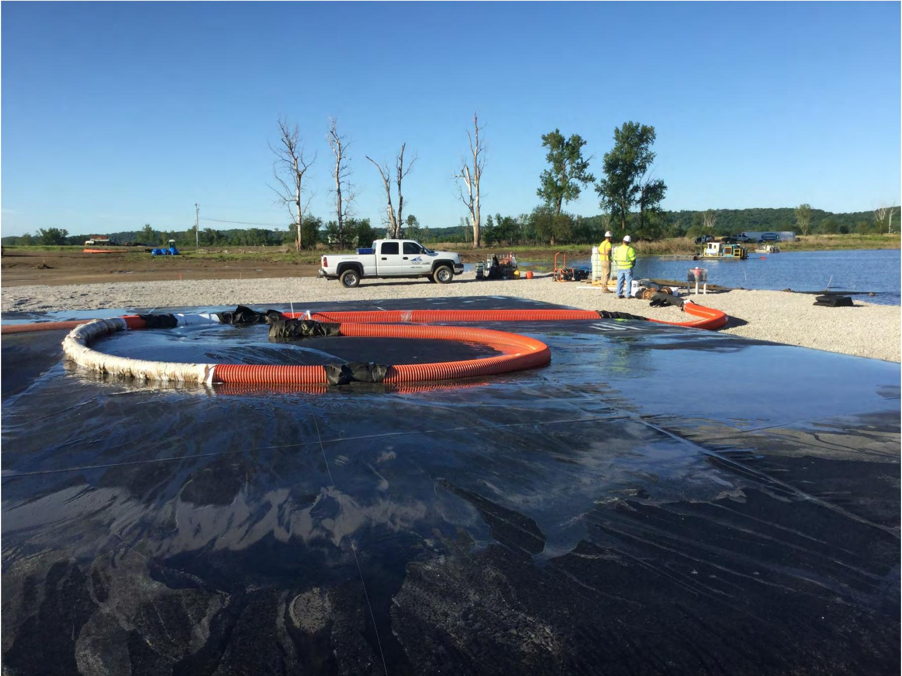
Figure 10: Iatan Ash Impoundment – installing geotextile tube system (east bank looking south)
