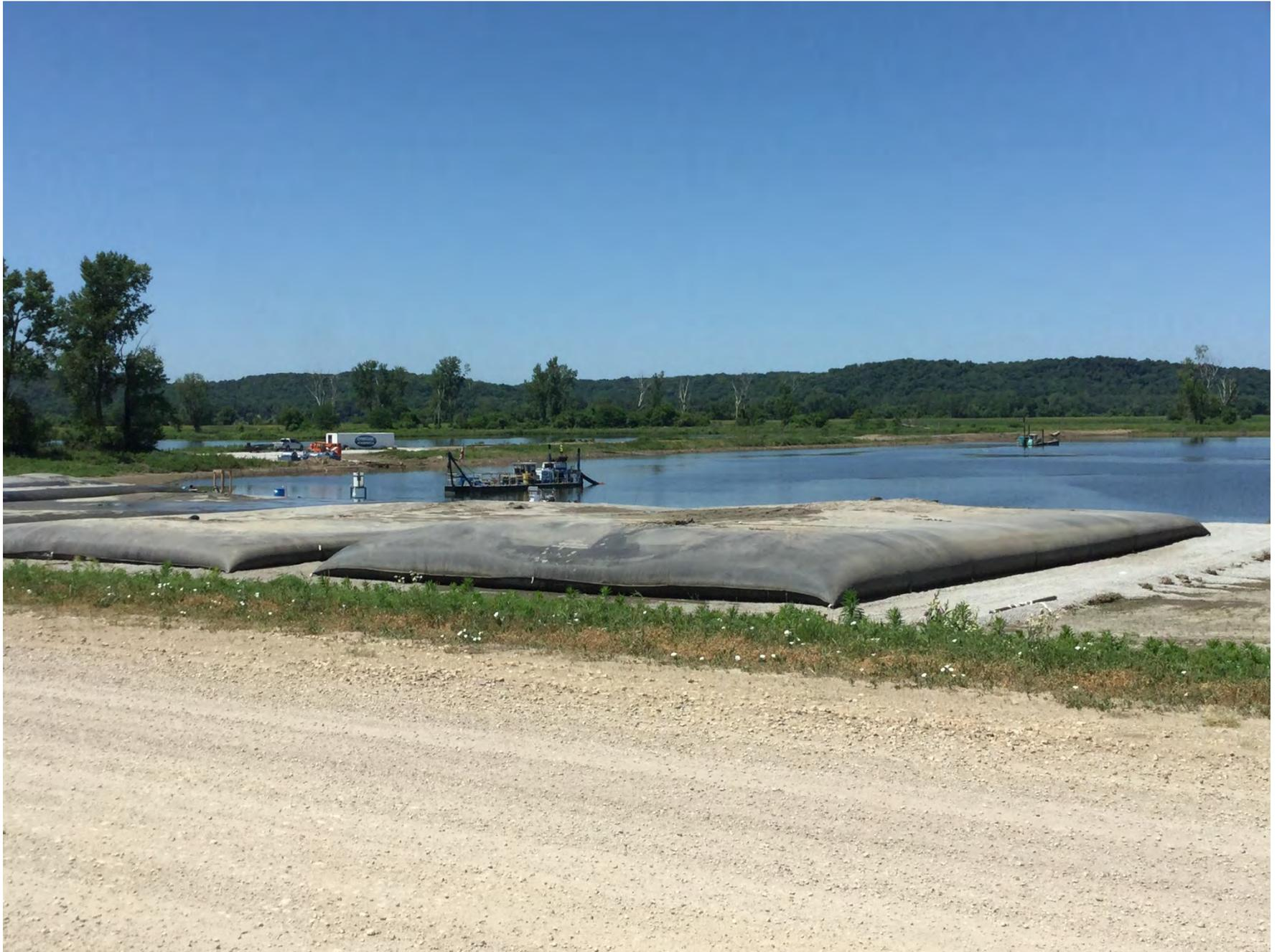
Figure 13: Iatan Ash Impoundment – filled geotextile tubes (east bank looking southwest)
