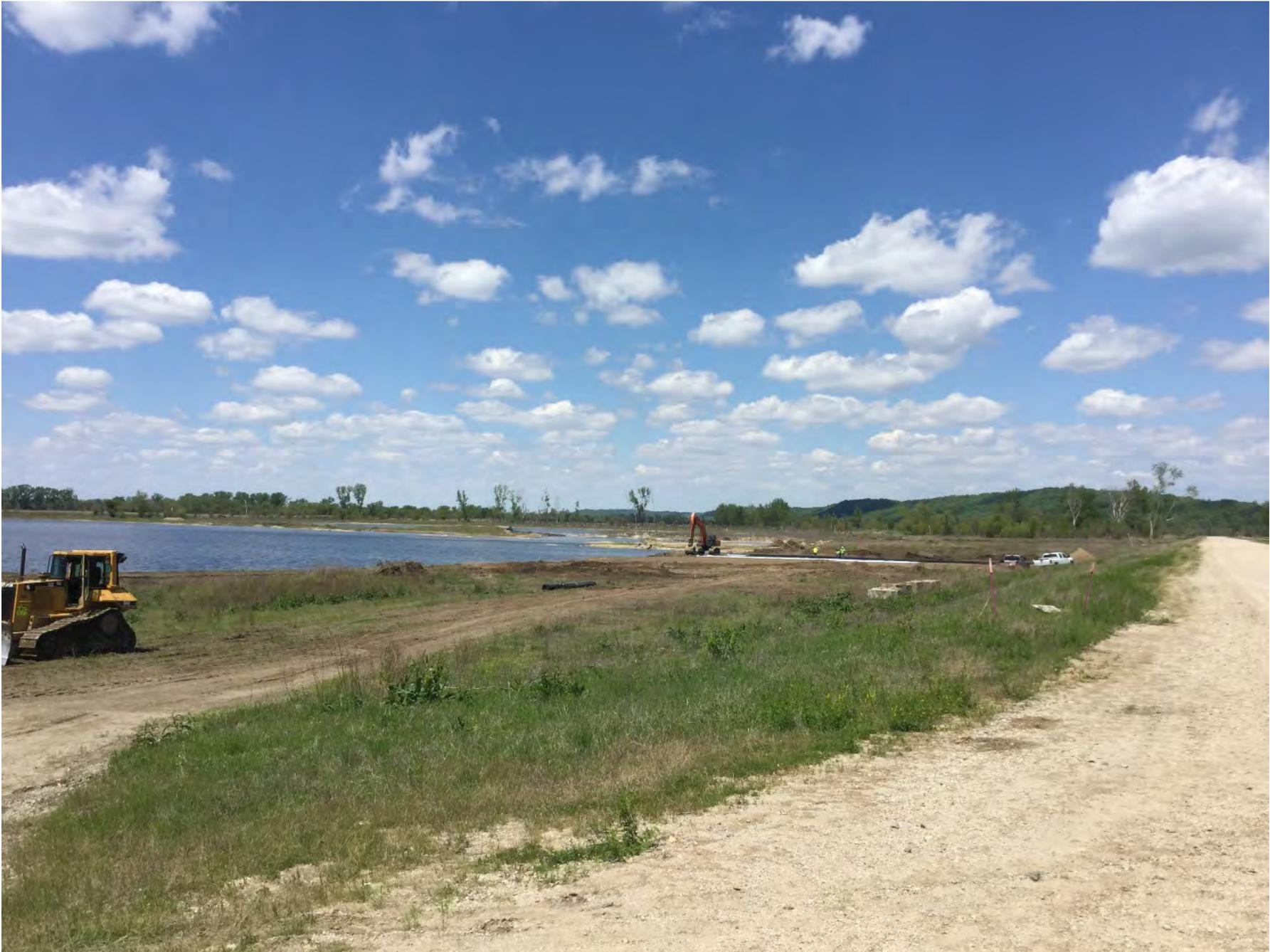
Figure 8: Iatan Ash Impoundment – prepping geotextile tube area (east bank looking north)
