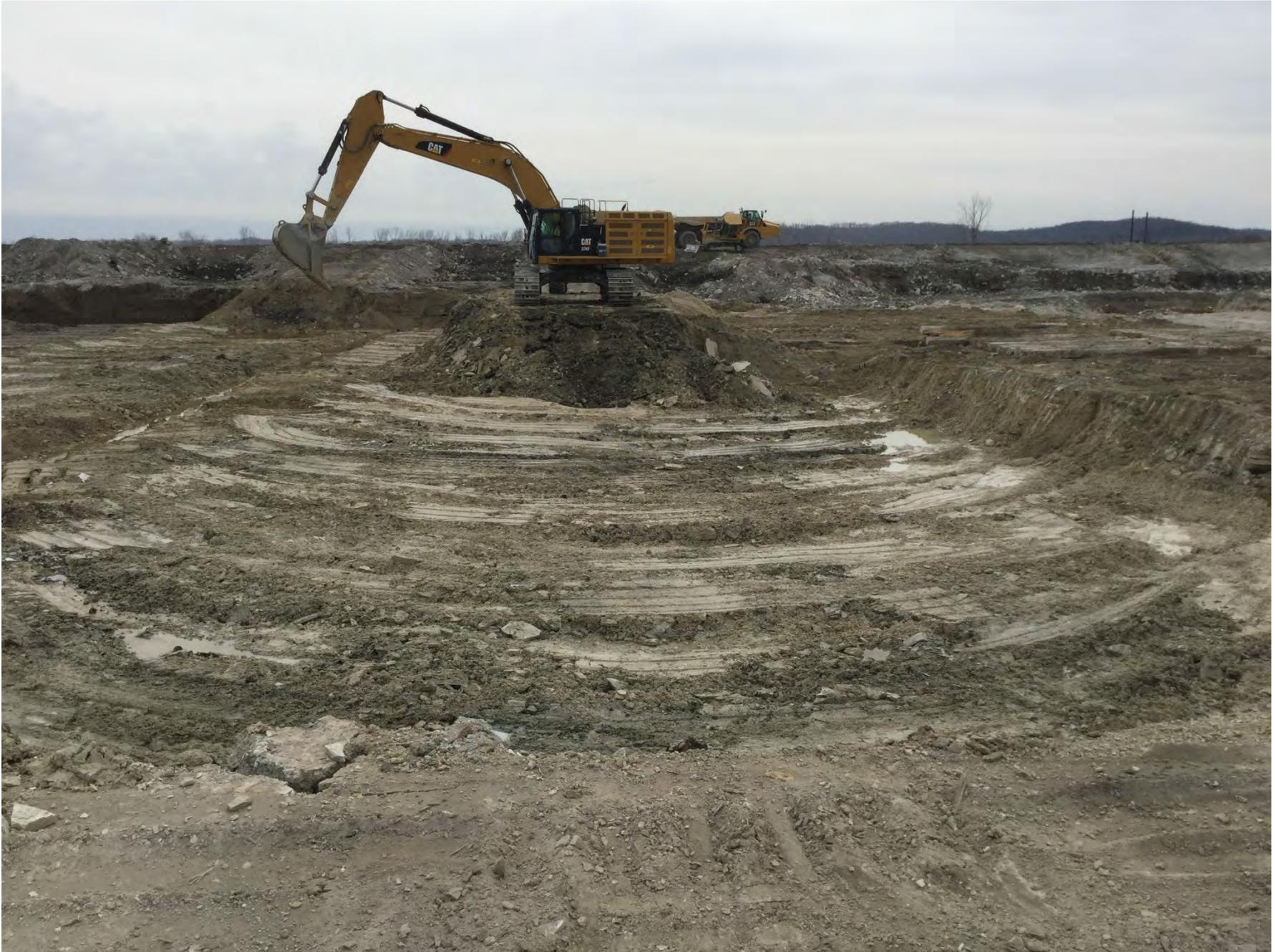
Figure 5: Iatan Ash Impoundment – mechanical excavation from north portion of pond (looking east)
