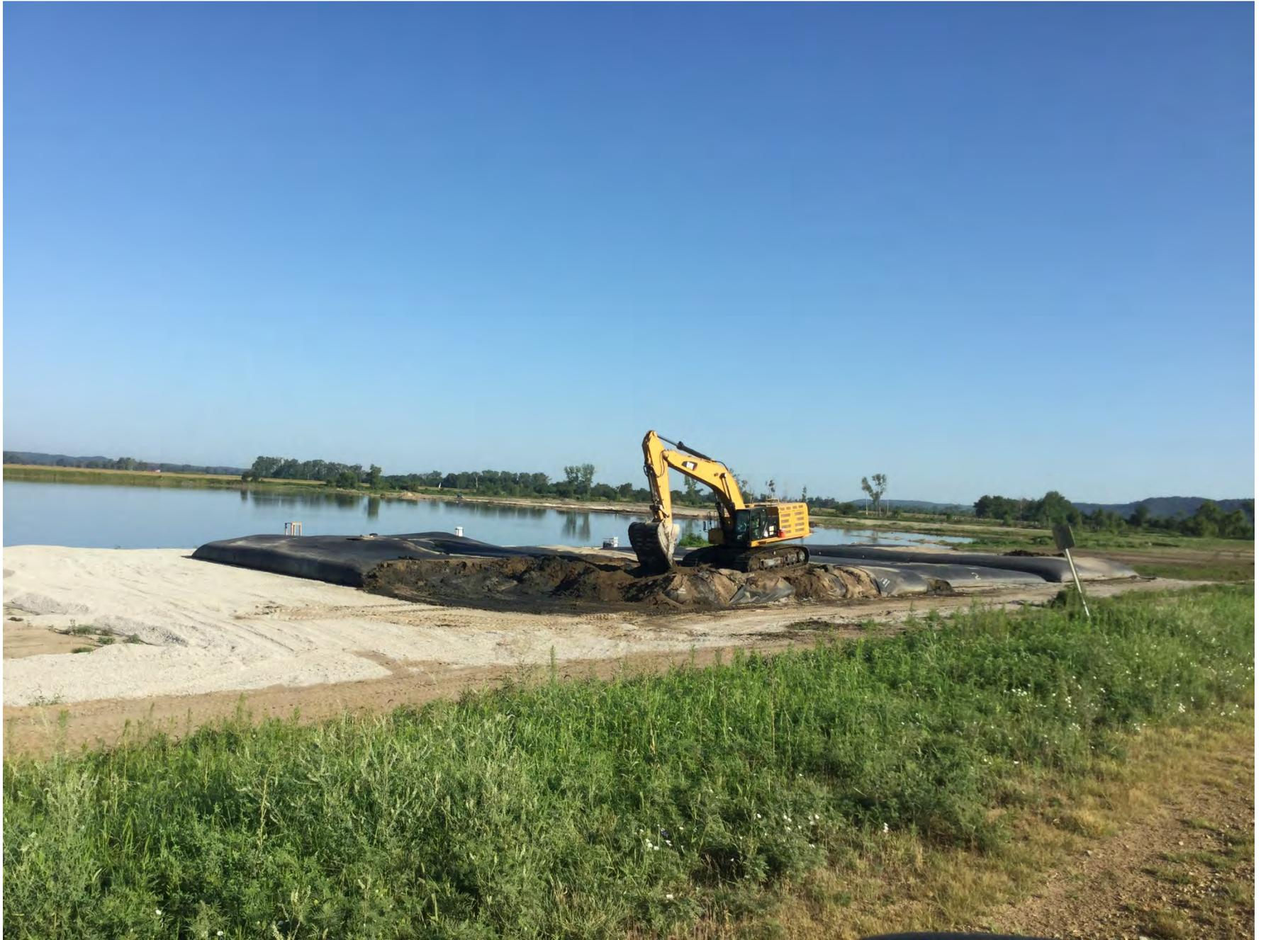
Figure 14: Iatan Ash Impoundment – excavating ash from geotextile tubes (east bank looking northwest)
