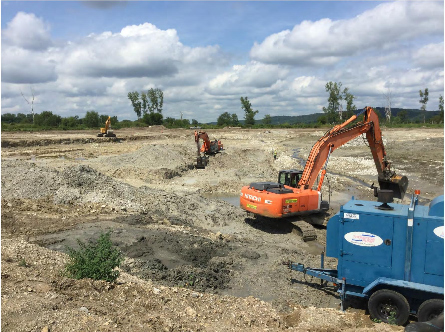
Figure 3: Iatan Ash Impoundment – mechanical excavation from north portion of pond (looking northeast)
