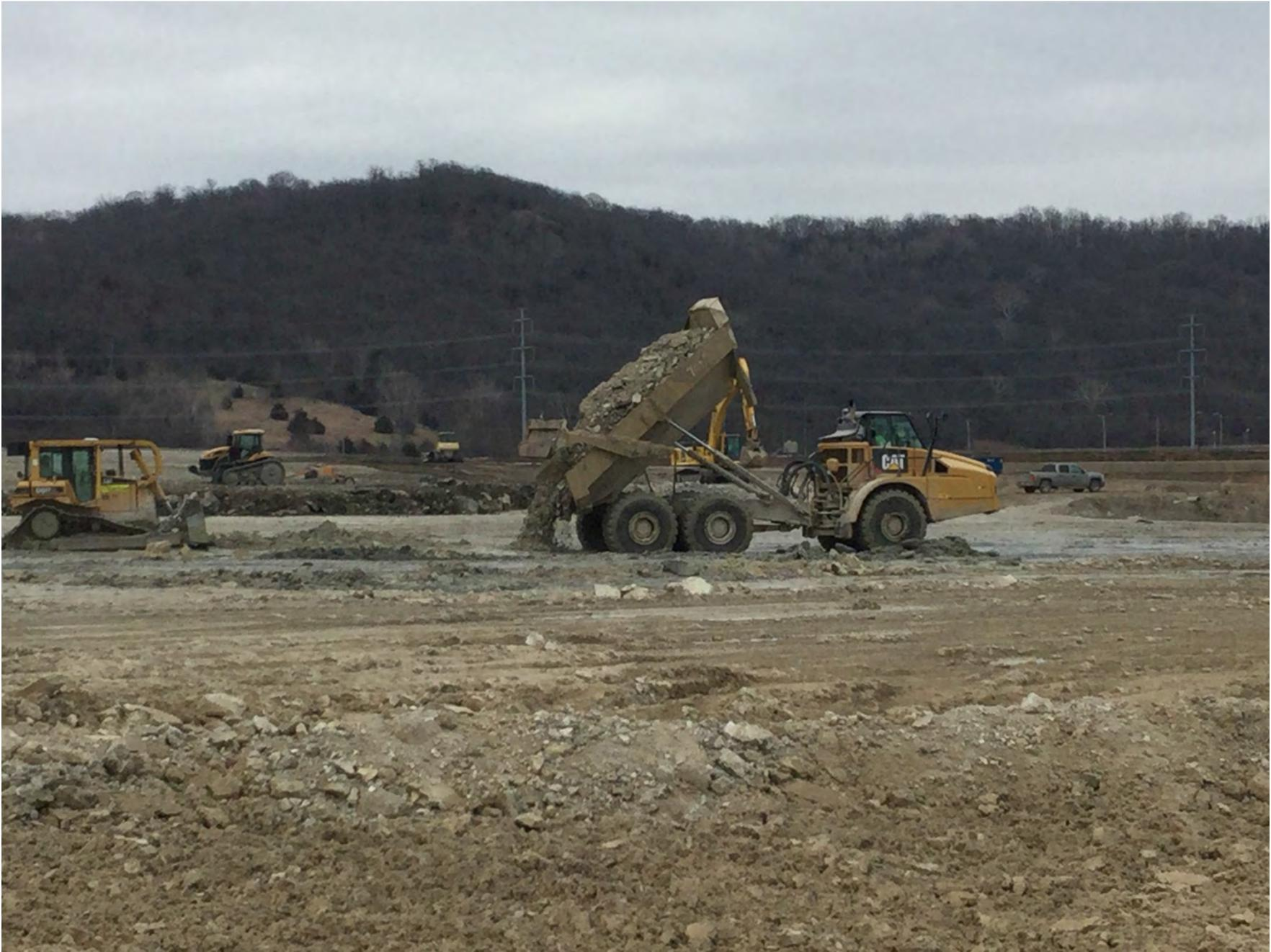
Figure 17: Iatan CCR Landfill – dumping excavated ash (looking east)
