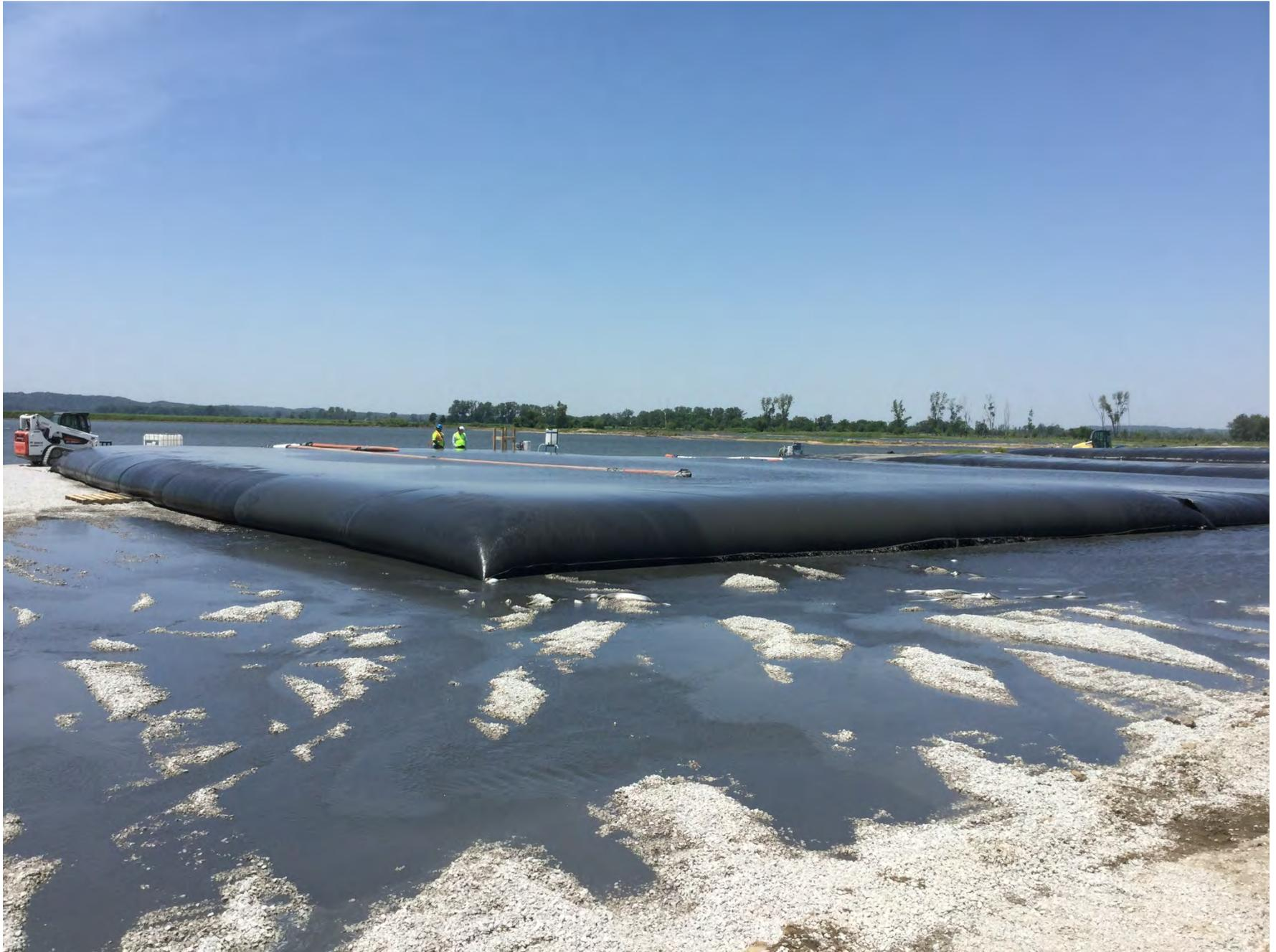
Figure 12: Iatan Ash Impoundment – filling geotextile tubes (east bank looking northwest)
